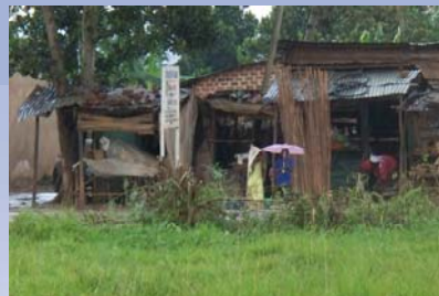
Infrastructure in need of restoration
